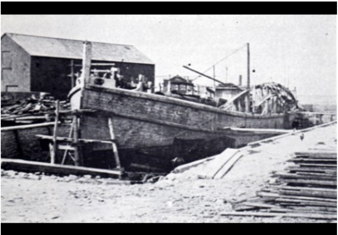
The City of Owen Sound being rebuilt in 1892 after 3 years on the bottom.
