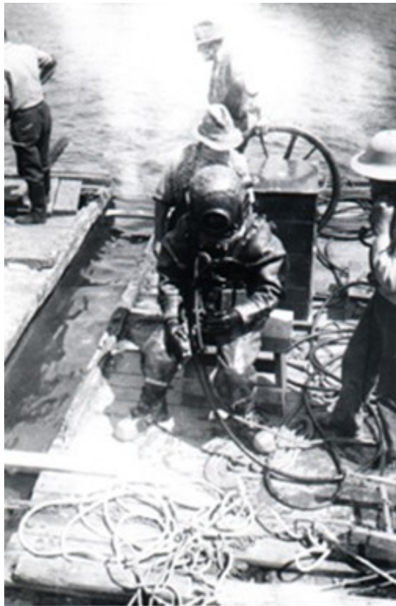
Divers prepare to descend 84 feet to the HIBOU that by 1942 was embedded in 7 feet of mud
